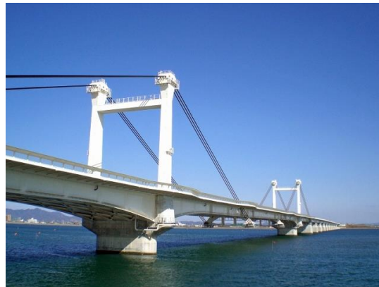
Cable stayed Bridge:Function separated type (girder+tower+cable+bearing+side wing+accessary) They are mainly fabricated and assembled at yard.
