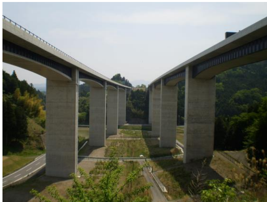
PC Bridge:Function integrated type (super structure+piers+side wall) They are constructed together at site.
