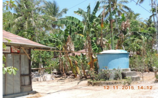
Figure 5 Rainwater harvested from roof-gutter
