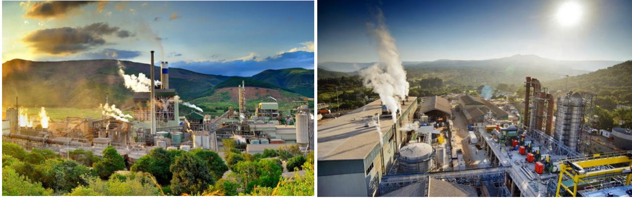
Exhibit 5. SAPPI Kraft Ngodwana Mill (Source: www.sappi.co.za).
