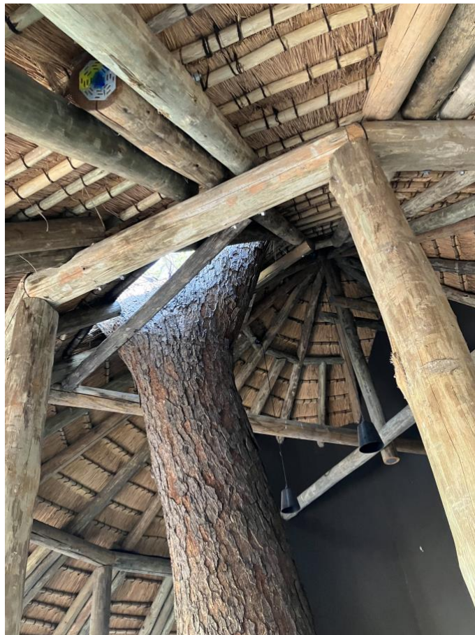
Exhibit 8. Skukuza airport baggage reclaim, underside of roof. Photograph by author.
