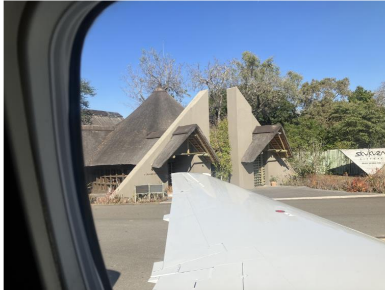
Exhibit 5. Skukuza airport terminal building, viewed from the window of an aeroplane after landing. Photograph by author.
